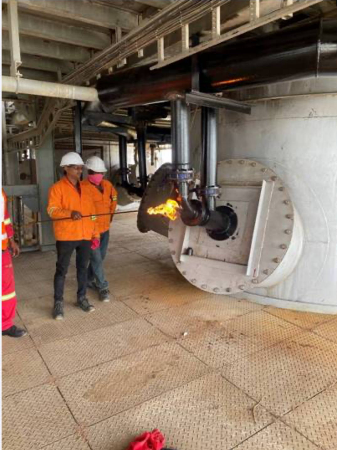
Figure 2: Successful firing of burners of Kiln 1 (12 February 2025).
