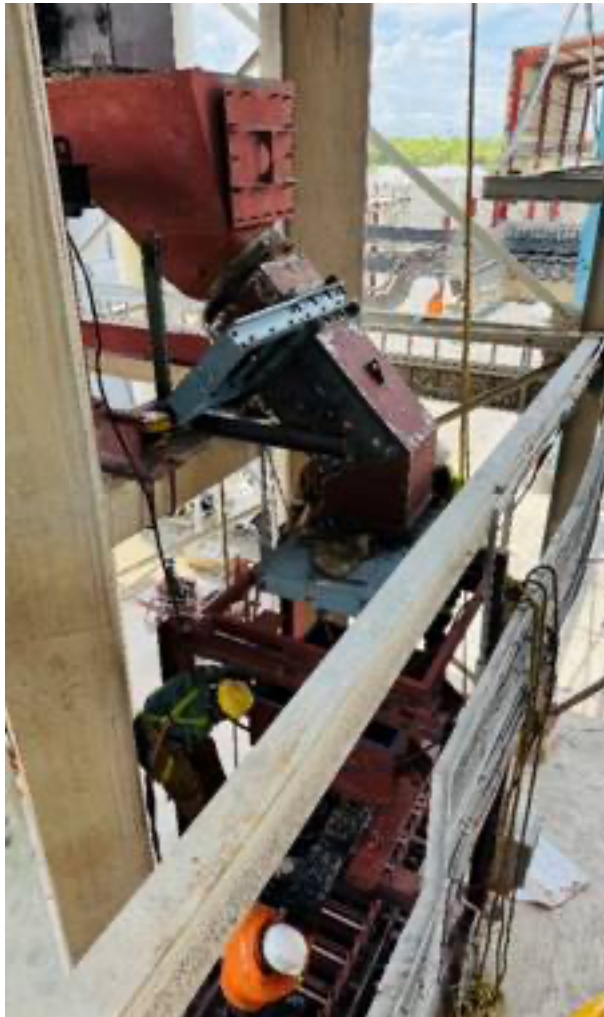
Figure 1: View of discharge and slide gates (left) and vibratory feeder above pan conveyor (right).
