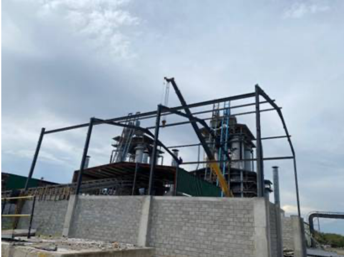
Figure 4: View of coal storage facility.
