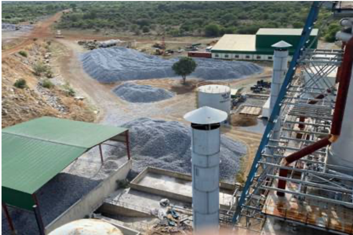
Figure 5: View of part of the kiln feed with lime plant in the background.
