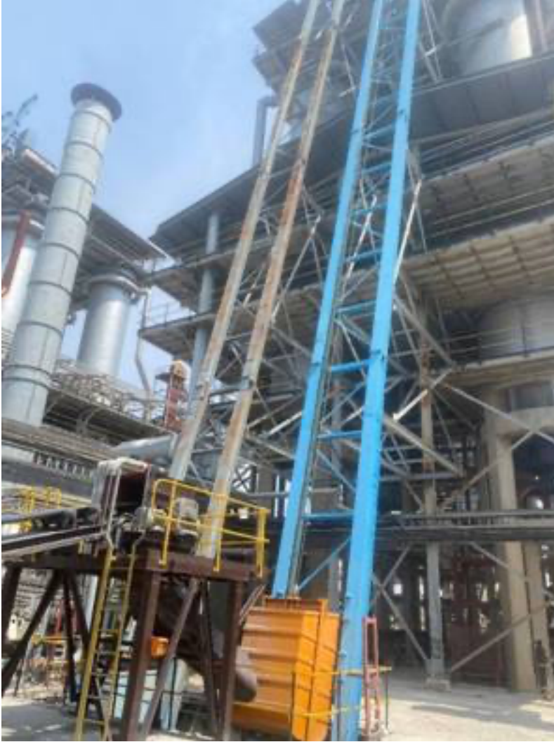
Figure 4: View of refurbished hoist structure (blue) and refurbished skip (orange).
