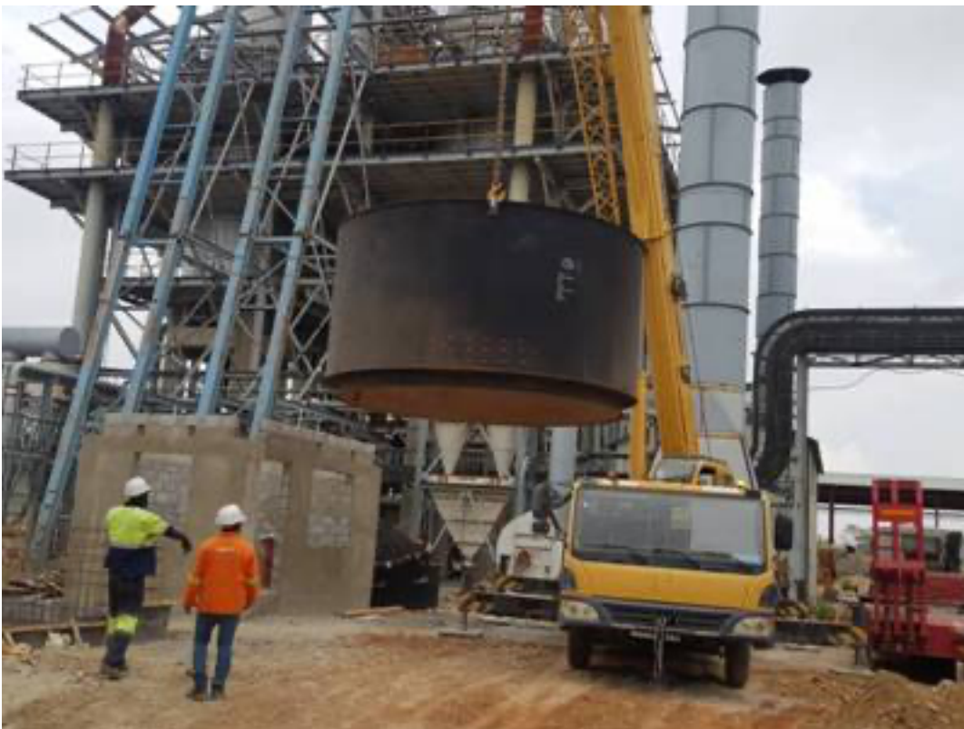
Figure 2: Parts of gasifier being off loaded at lime plant, 29 October 2024.
