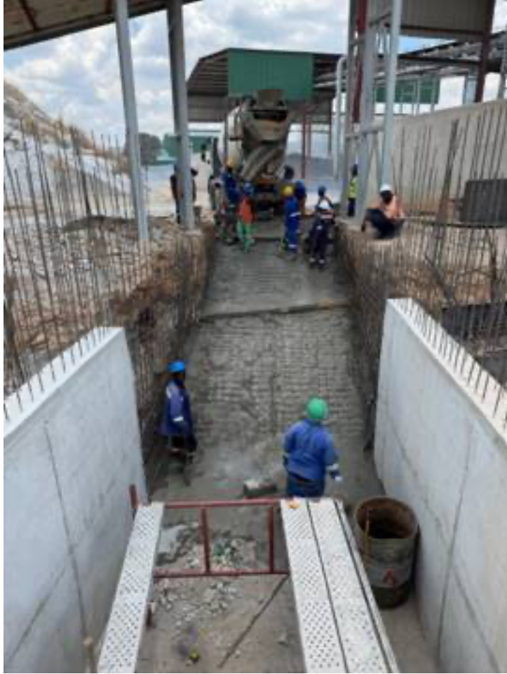
Figure 5: View of incline ramp from coal storage facility to coal gasifier.
