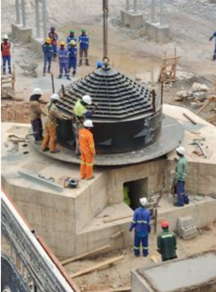
Figure 3: Erection of gasifier
