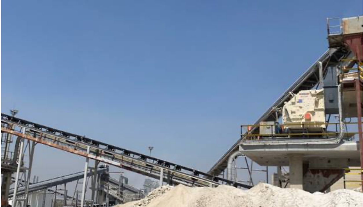
Figure 5: View of the newly installed impact crusher.
