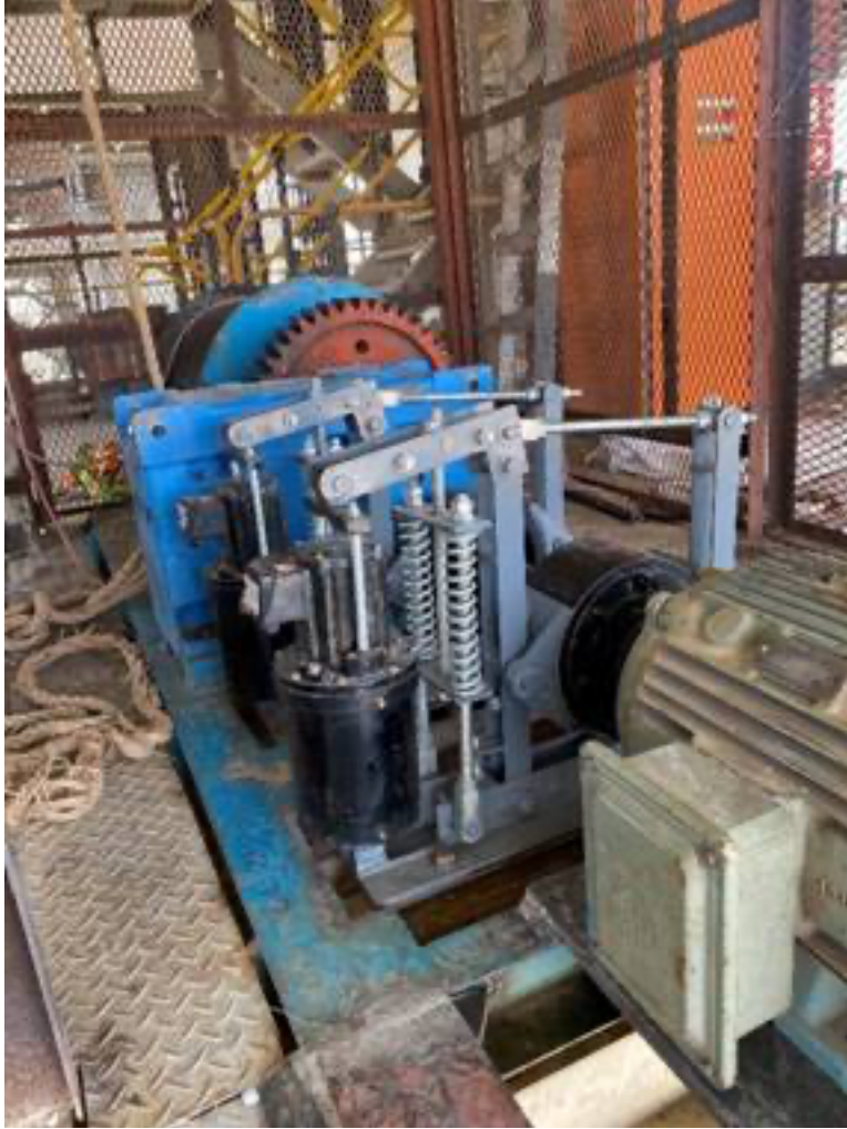
Figure 2: View of newly installed brakes for the skip hoist motor.
