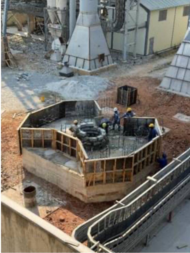
Figure 3: Preparation work at gasifier foundation ahead of final concrete pour.
