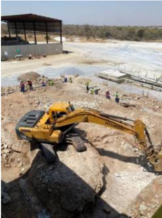
Figure 4: View of excavation work at coal storage facility.
