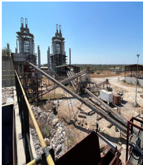
Figure 2: Primary crusher with lime plant in background (Source: Limeco, 2023).
