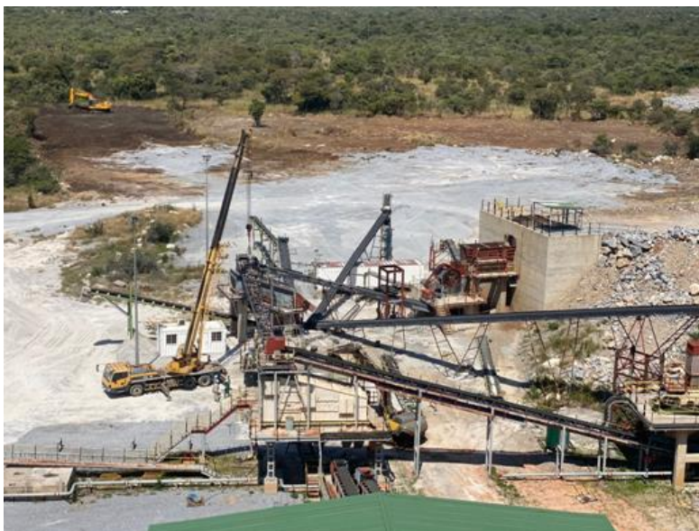
Figure 4: Aerial view of renovations at crushing plant (Source: Limeco, 2024)
