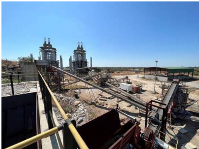
Figure 1: View of plant from primary crusher
